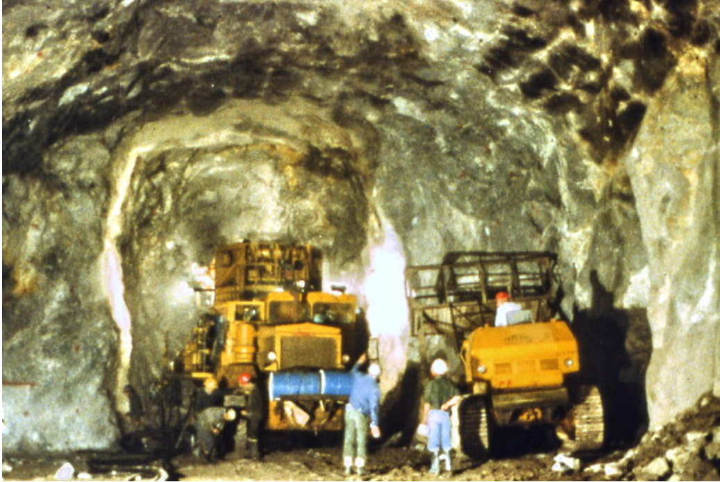
Figure 4: A 6 m wide heading driven ahead of the tunnel face to permit pre-reinforcement of potentially unstable wedges in the roof. The seven-boom jumbo is seen working in the heading.
